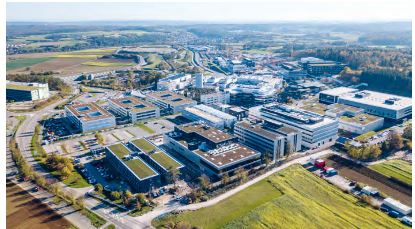
THE WEISSACH DEVELOPMENT CENTRE
